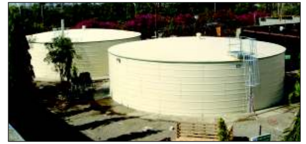
▶ Over 1.5 million Ltrs. Installed at ITC Pune, India
